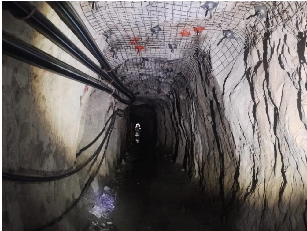
Figure 6 – Back height increased in the Amalgamated Adit to hang the High Voltage 11kV cables and services.
