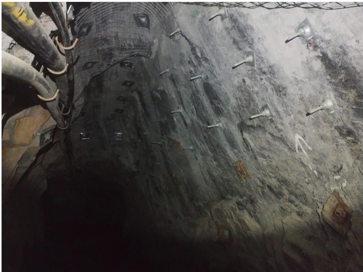
Figure 3 The underground substation cuddy completed
