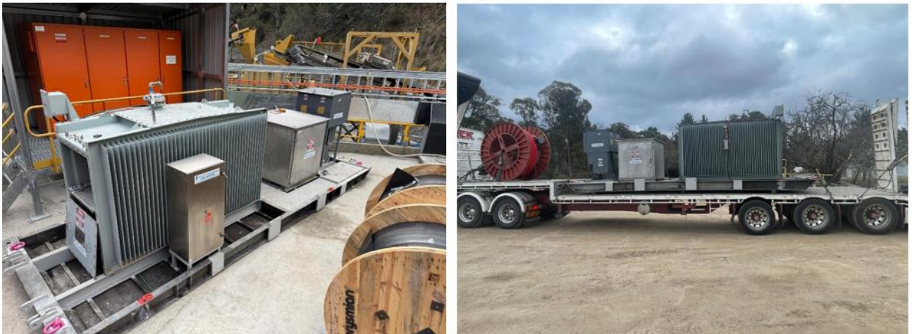
Figure 1 – High voltage (415V to 11kV) transformer installed next to power station at the Reward Gold plant
