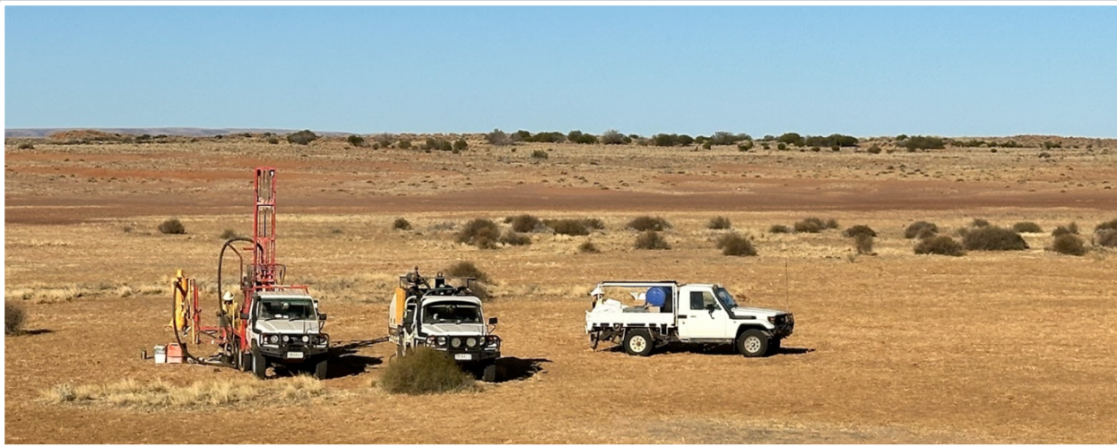
Figure 1. Low environmental footprint, Toyota mounted air-core drill rig on Nilpinna EL7071, making rapid progress.
