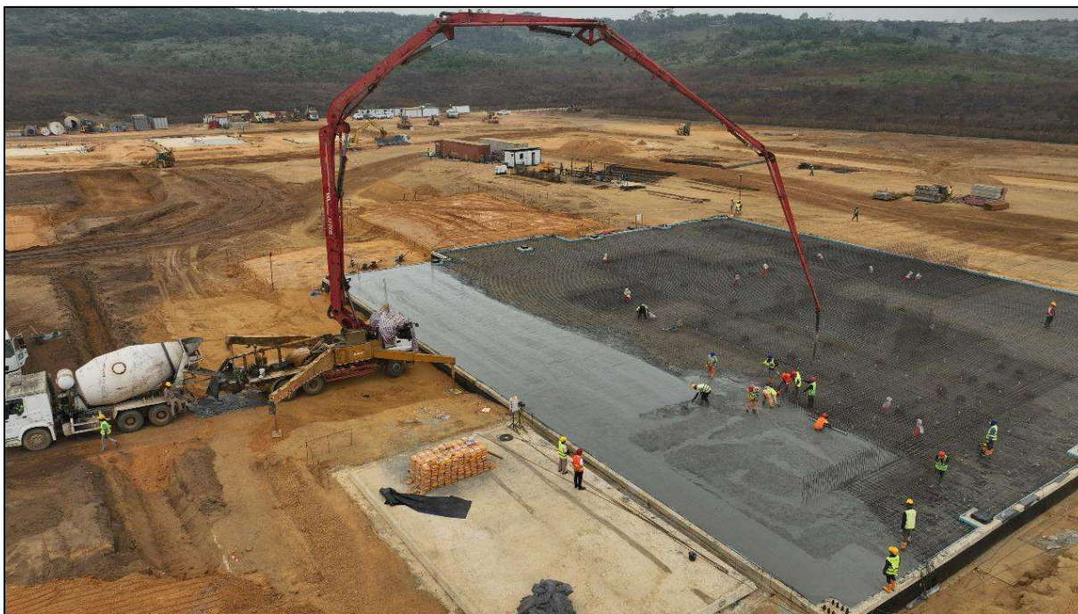
Figure 2– Subantando Fertilizer Plant, located in Cabinda, Angola – concrete pour for the slab underway.
