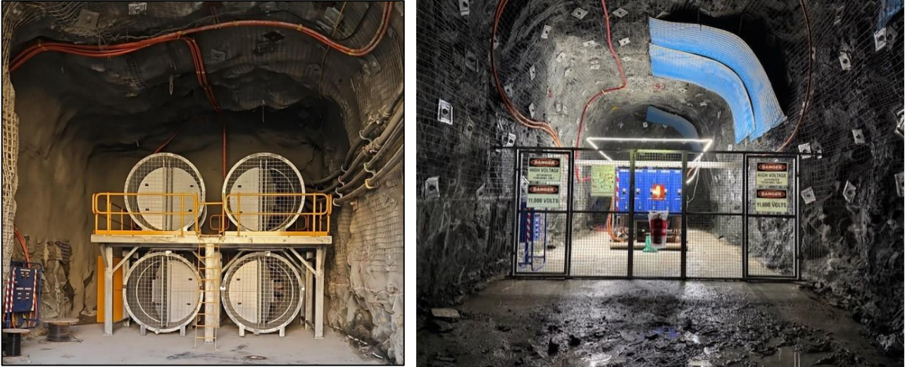
Figure 8 & 9: Never Never underground primary fan installation and first underground electrical sub-station
