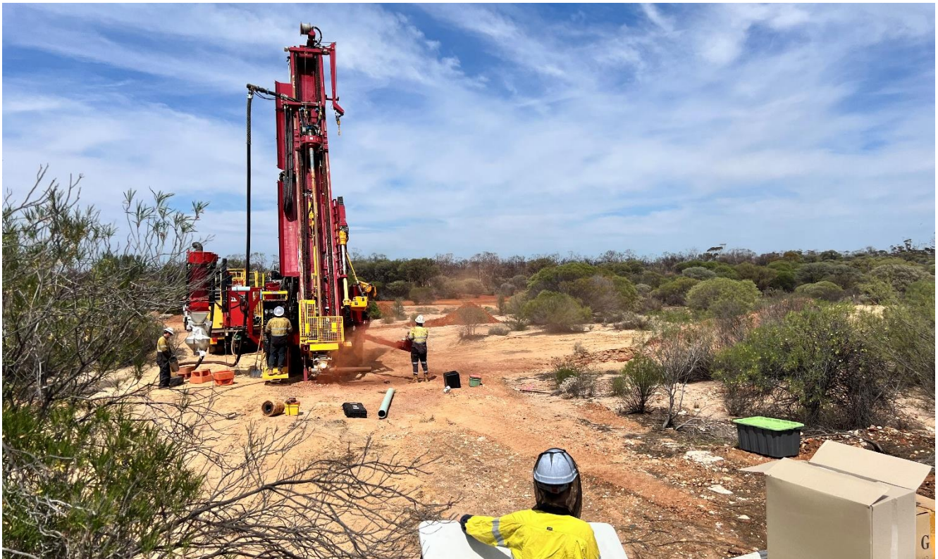
Figure 1 Frontline Drilling rig at Cheer Prospect, Comet Vale
