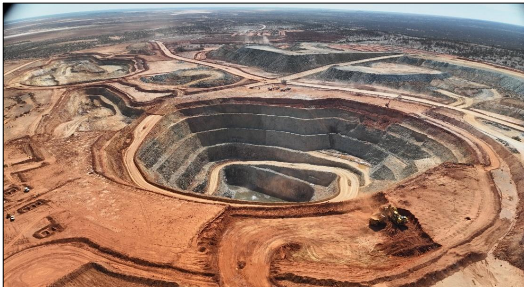
Cue open pit mining – Break of Day Stage 2 (facing North)
