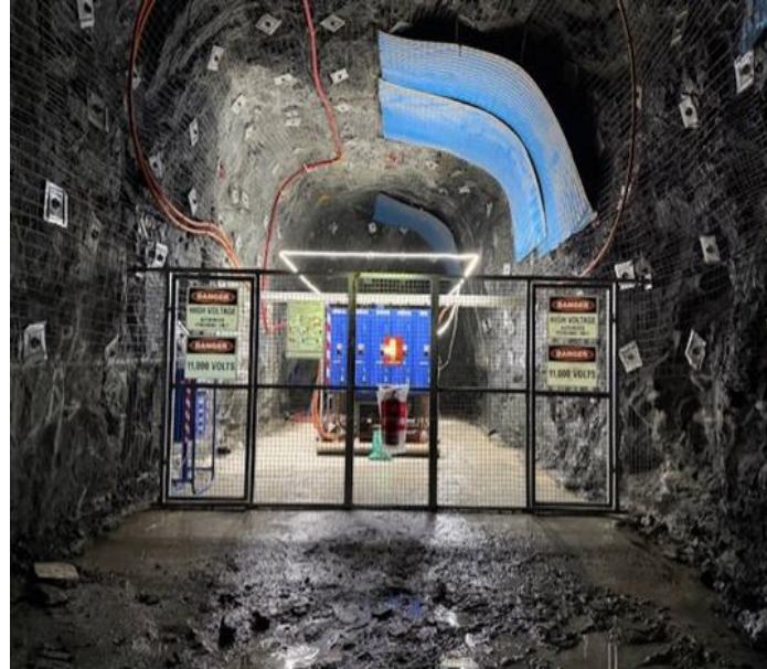
Never Never underground primary fan installation and first underground electrical sub-station
