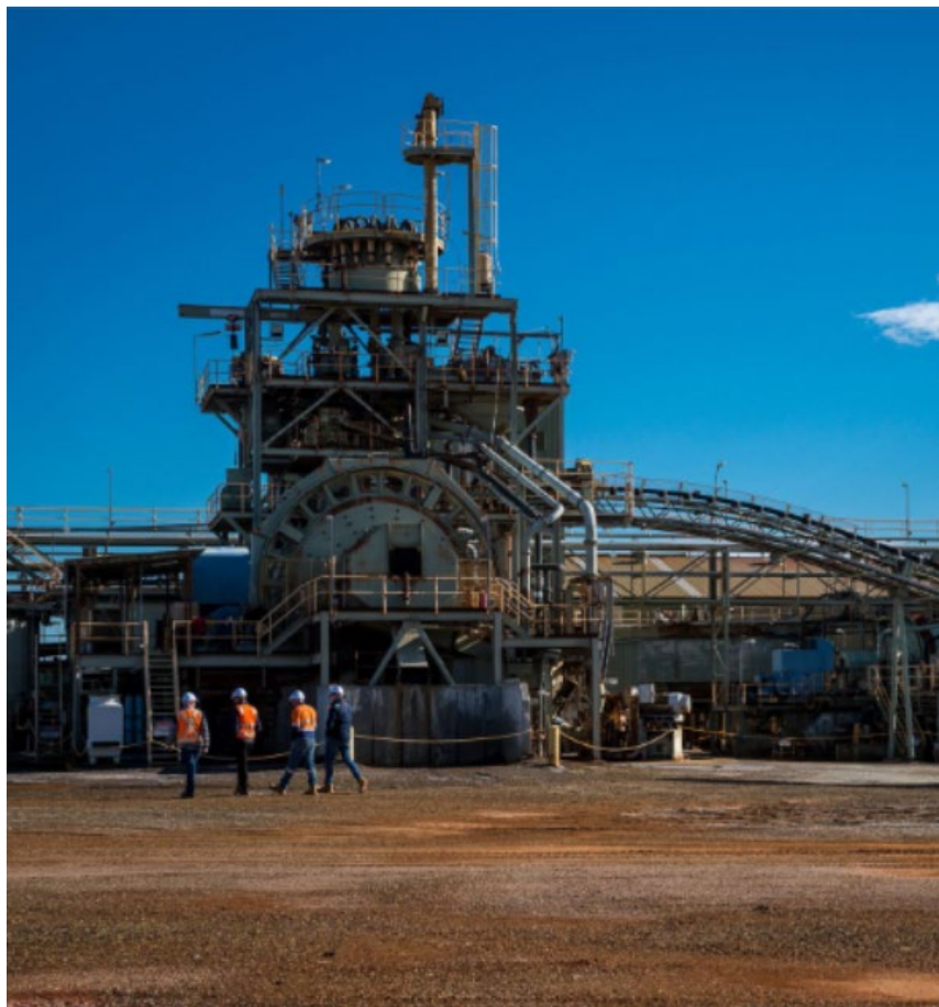
Figure 2. Lake Johnston processing plant.
