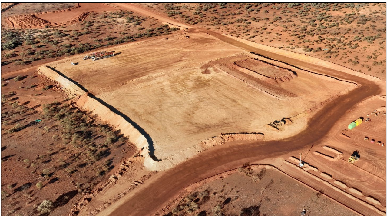
Figure 5 – Ore Stockpile being built on ROM
