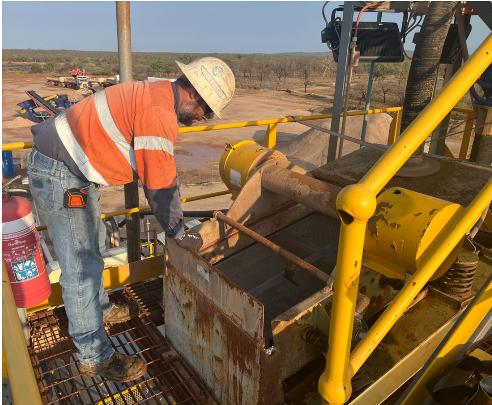
Figure 2: replacing the nelson scalping screen mat
