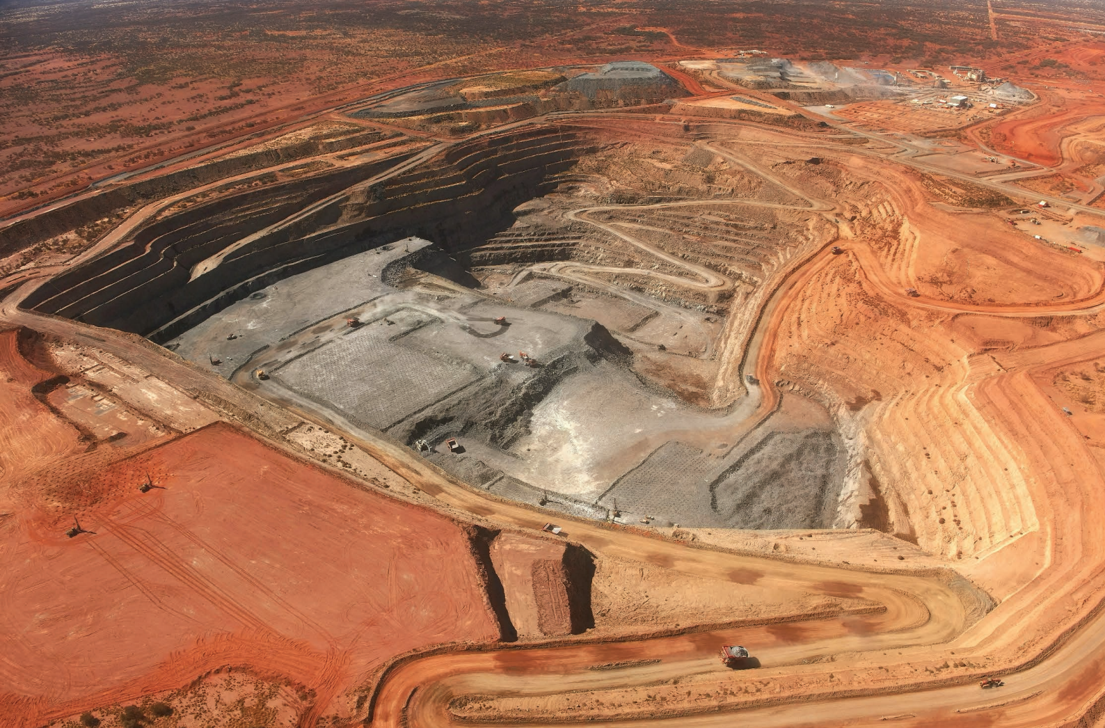
Karlawinda Gold Project – Bibra open pit (June 2025)
