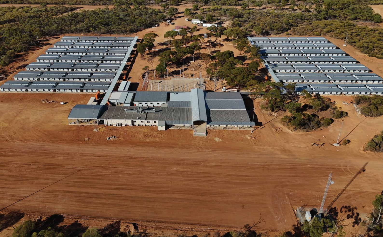
Mt Gibson Gold project – accommodation village installation
