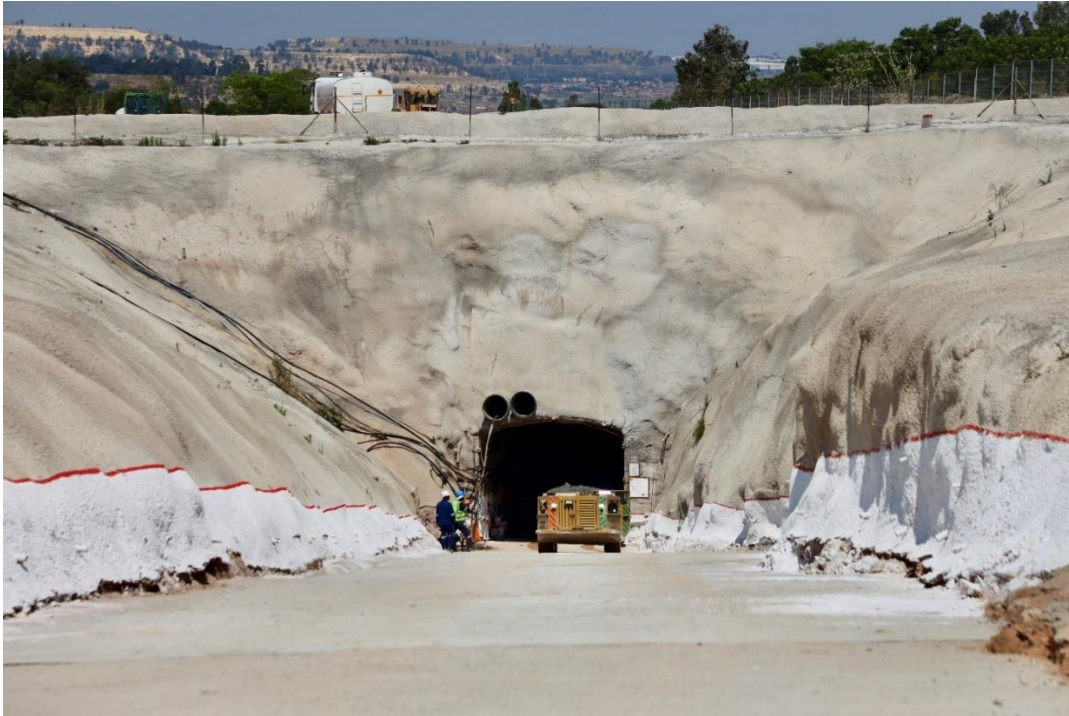
IMAGE 5: LHD EXITING QALA SHALLOWS CONCRETED BOX-CUT ROADWAY WITH THE FIRST LOAD OF ORE
