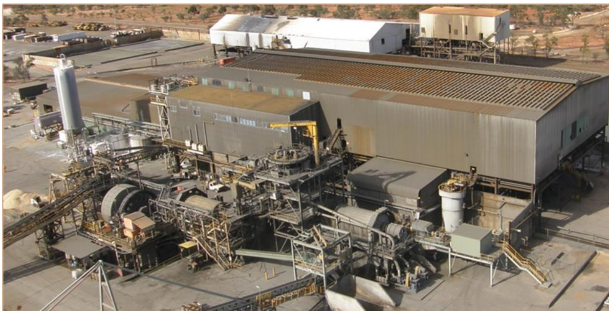
Figure 2: Endeavor Mine Processing Plant
