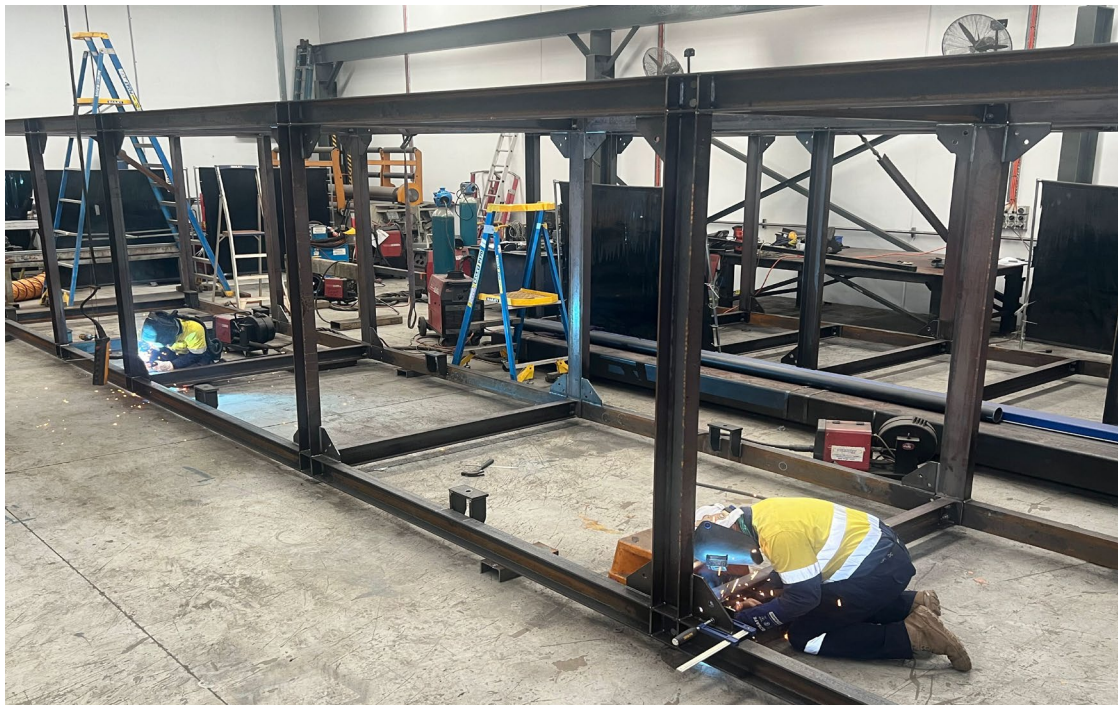
Figure 3. Structural steelwork for nano-filtration skids
