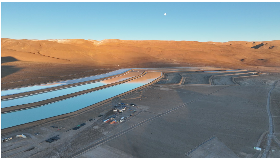
Figure 1. HMW Phase 1 evaporation ponds
