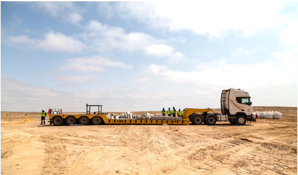
Figure 3: Local Namibian contractor, Tulela Mining & Construction, establishing onsite ahead of commencing the heap leach drainage material blasting.
