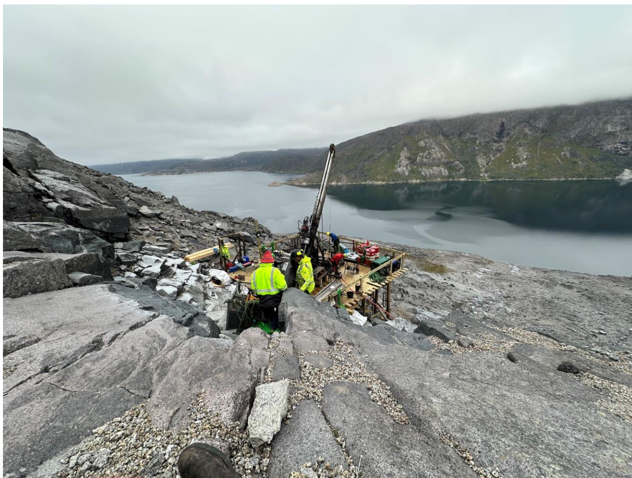
Figure 5 Drill Pad 25-7 with drill holes 25-7, 25-7A, 25-7B, 25-7C on 4 different azimuths
