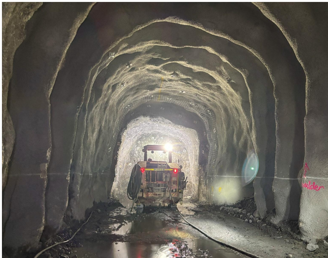
Figure 4. Upper North Lode high grade silver 10100 development drive.
