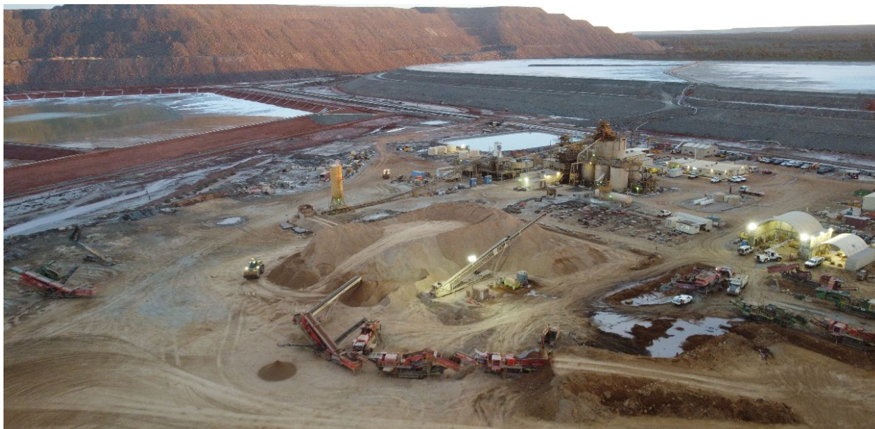
Figure 11: Lakewood Processing facility
