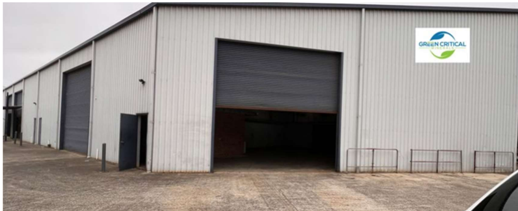
Figure 1 - GCM VHD Technology Industrial Facility
