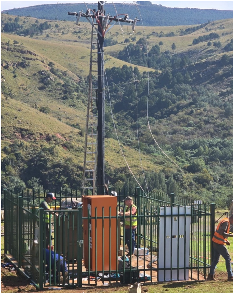
Figure 2: Installation of temporary electrical plant supply
