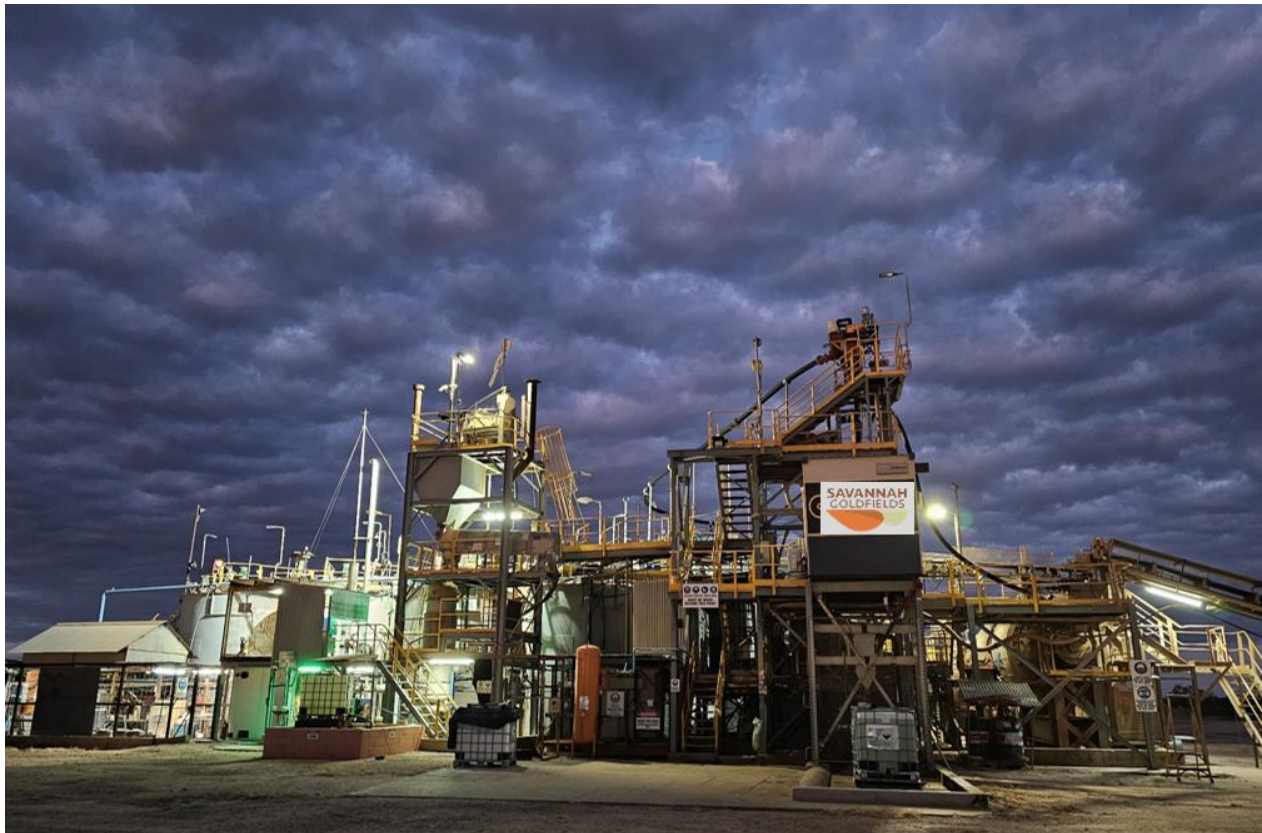
Georgetown Processing Plant
