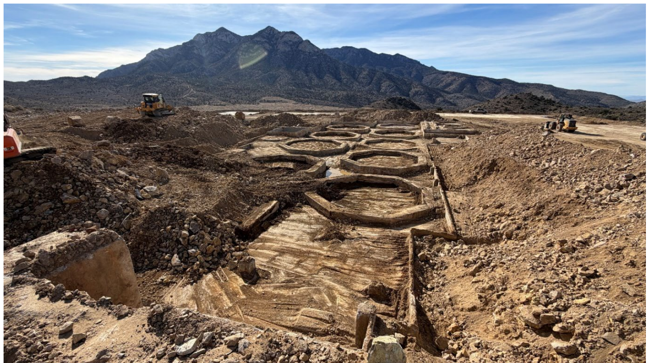
Figures 2: Uncovered concrete structures at Colosseum
