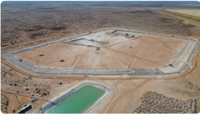
Photo 6: 13ha Water Storage Dam on 65ha TSF footprint.
