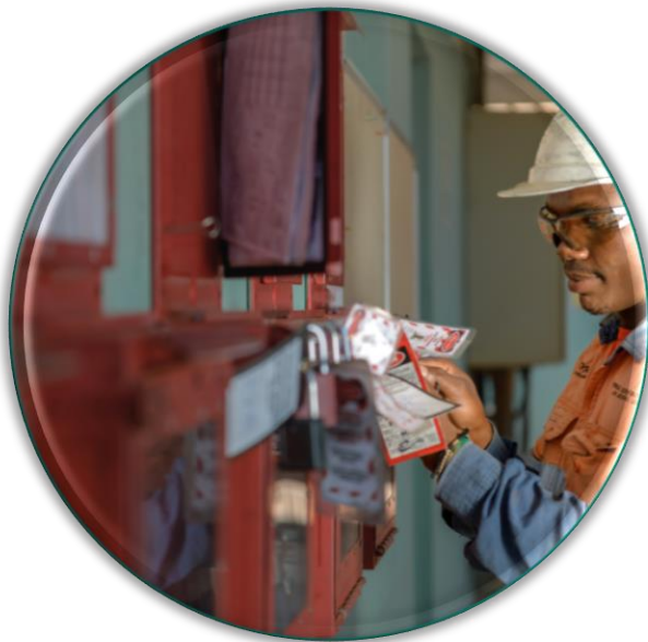
Lockout / Tagout inspection
