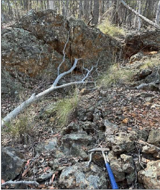
Figure 1 – Vertical shaft/stopes. Located at 710894E, 6259083N.
