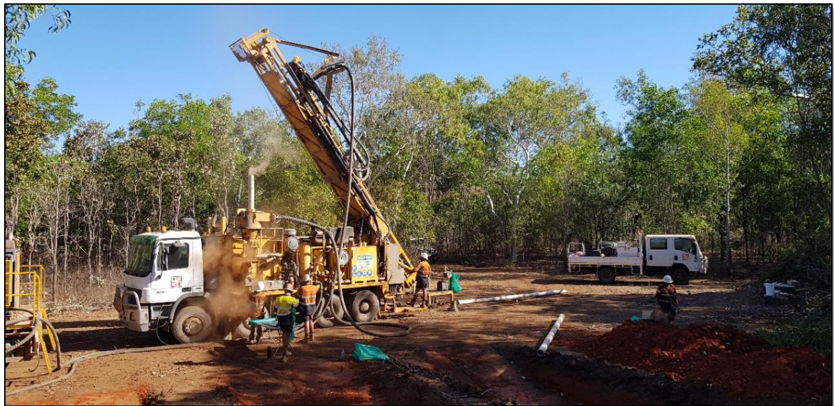
Figure 1 - Fenton Gold Project, RC drill rig undertaking pre-collar work, located in the Northern Territory.
