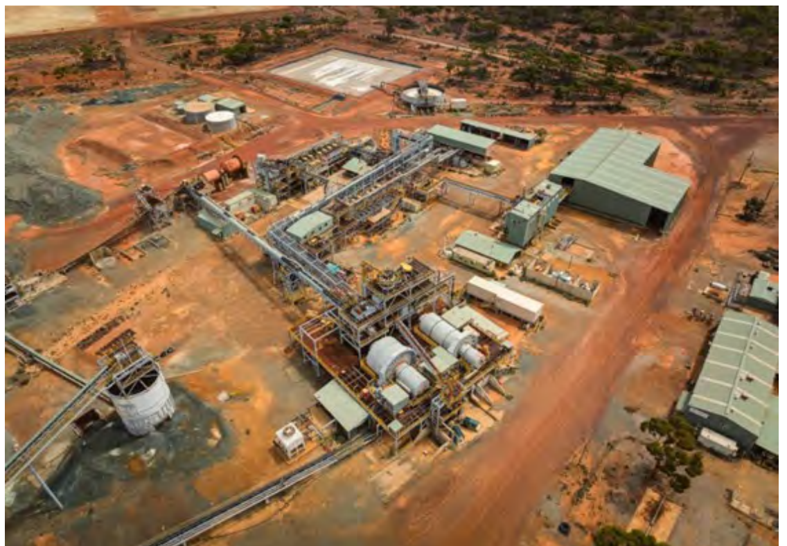
Figure 2: Black Swan processing plant
