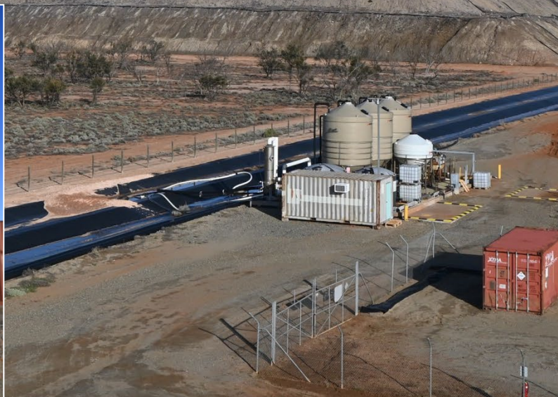
HDPE Liner arriving on site
