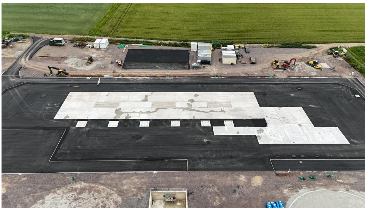
Figure 12 Aerial shot of the Phase One Schleidberg
