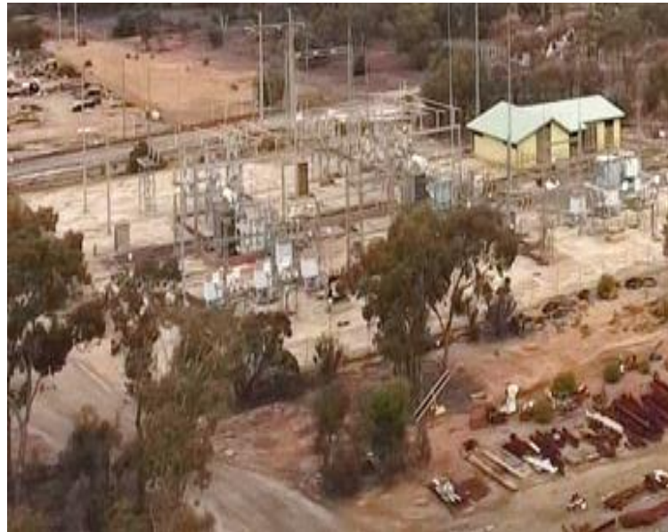
Grid power 15 MW / 132 kV, sub-station owned and maintained by Essential Energy.
