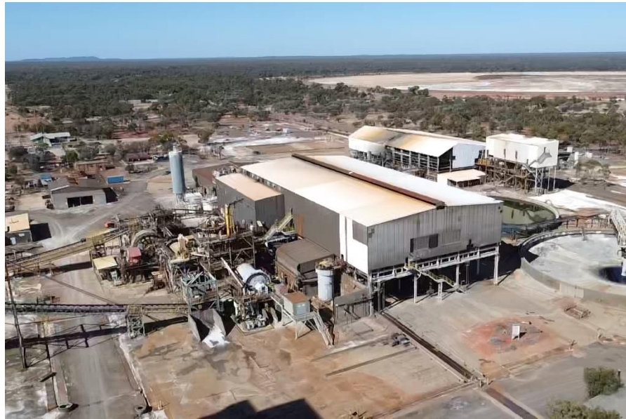
1.2 MTPA processing plant including a surface crushing plant, SAG mill, two ball mills & Pb/Zn flotation circuit.
