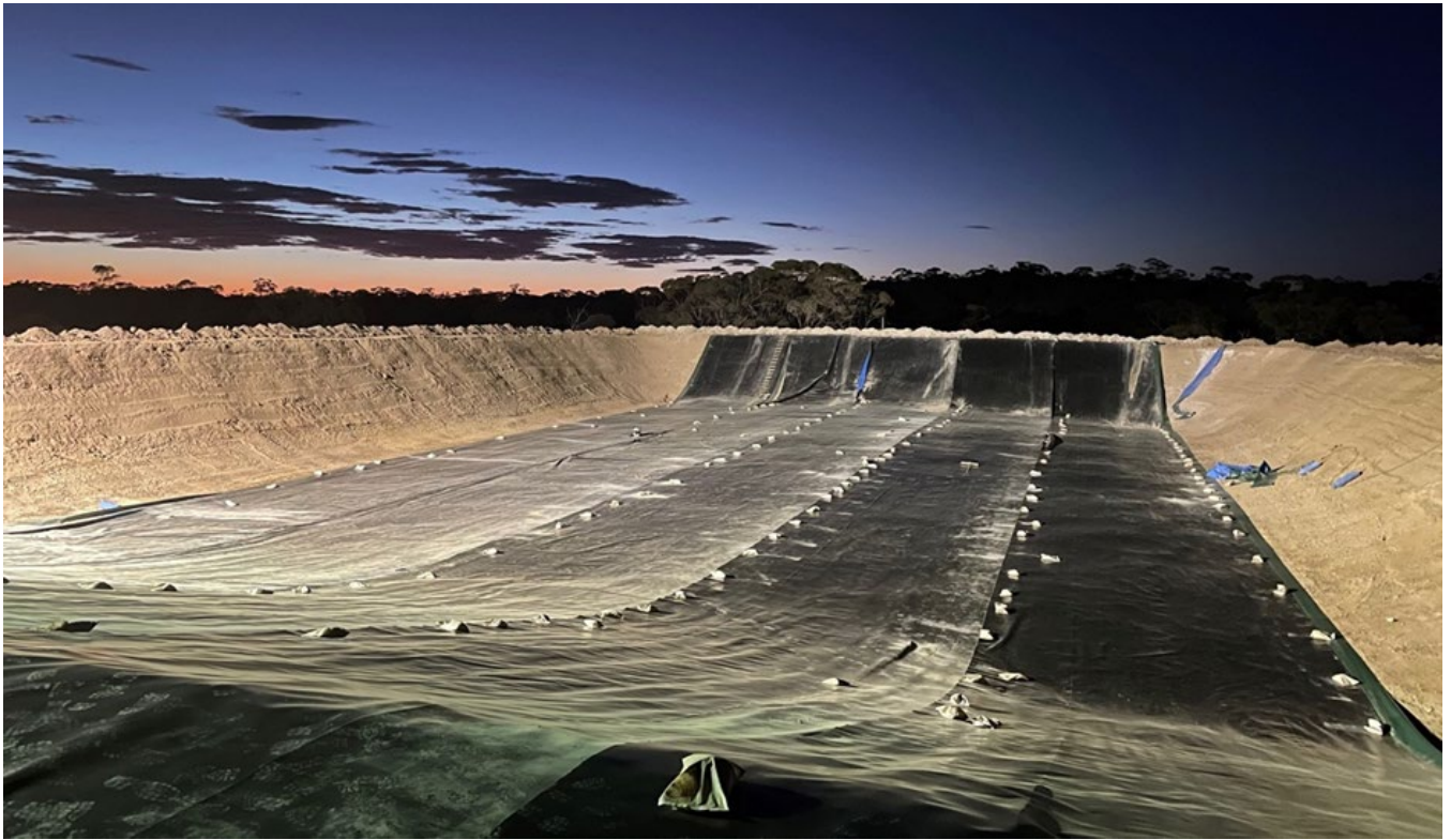
Figure 1: An Eastern Goldfields example of a vat leach pad under construction (source: Vat Leach Consultant)
