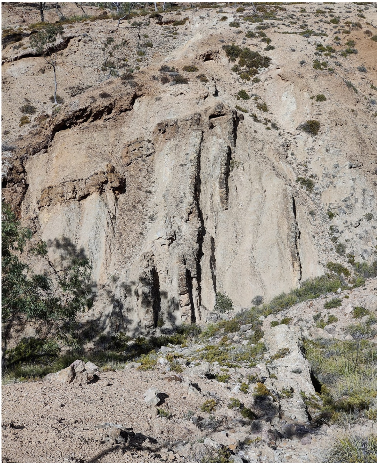
Figure 7. Vertical bedding parallel shears exposed by deep erosion gullies
