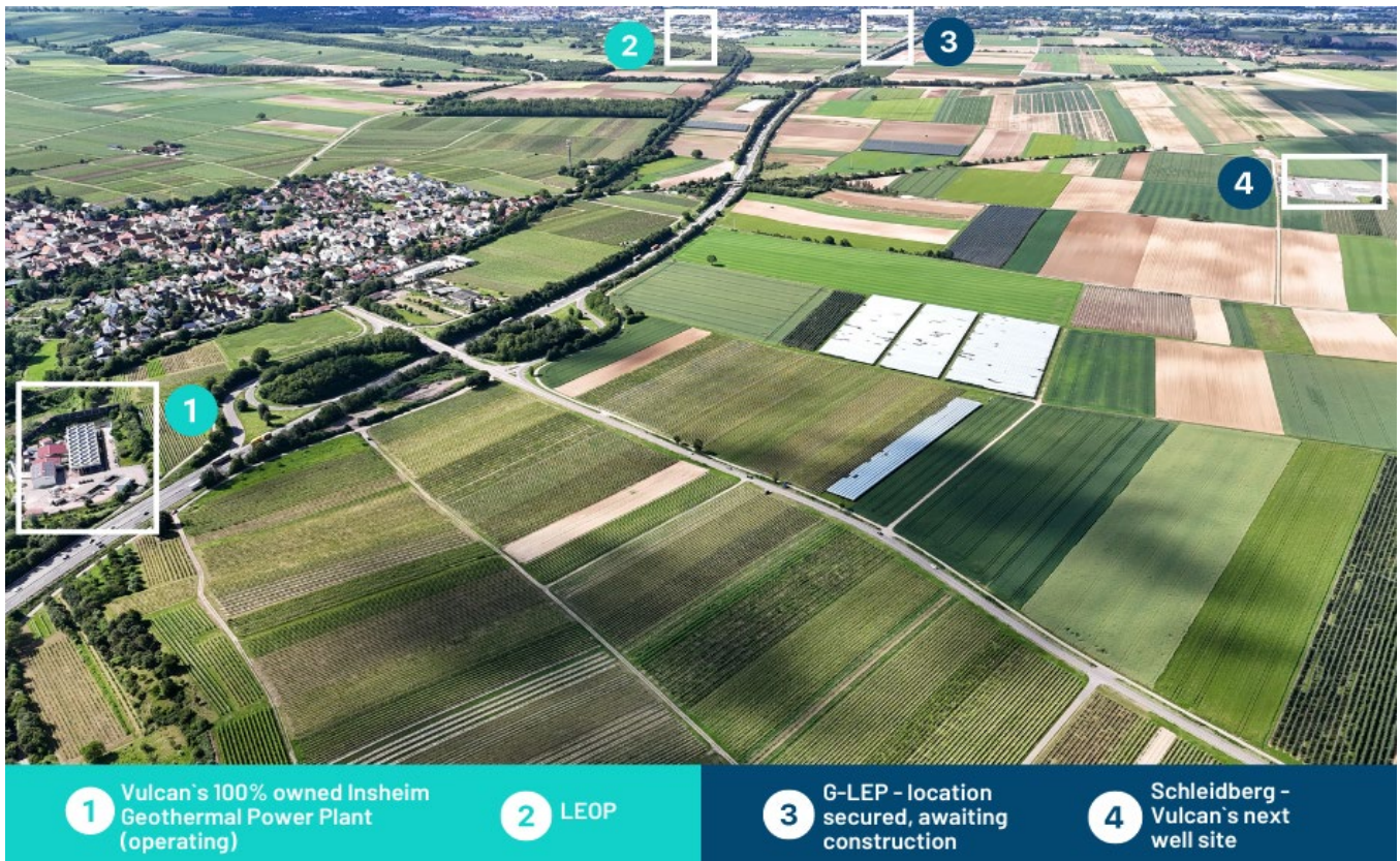
Figure 1 Aerial shot of part of Vulcan's upstream Phase One area in the Landau region, including the Natürlich Insheim geothermal renewable energy wells and plant, location of the LEOP, commercial G-LEP and the Schleidberg well site.
