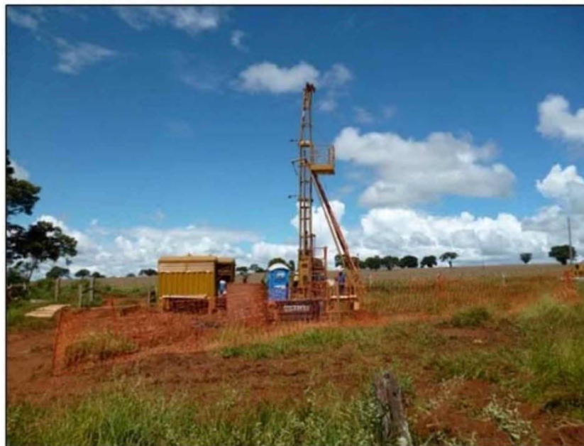
Figure 6-5 – Drilling equipment in operation in borehole PMC-FD-0074
