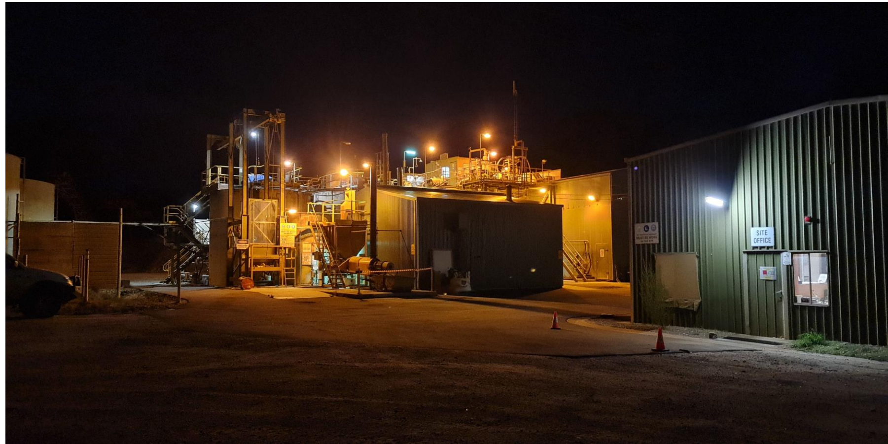
Maldon Processing Plant
