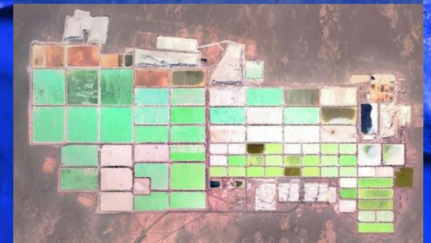
Multiple Evaporation Operations
