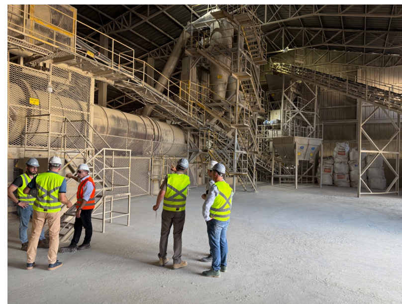
DB Processing Plant – Rotary Kiln
