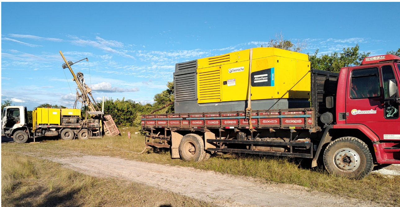
Photo 2: Drill rig advancing inclined Hole RC-011
