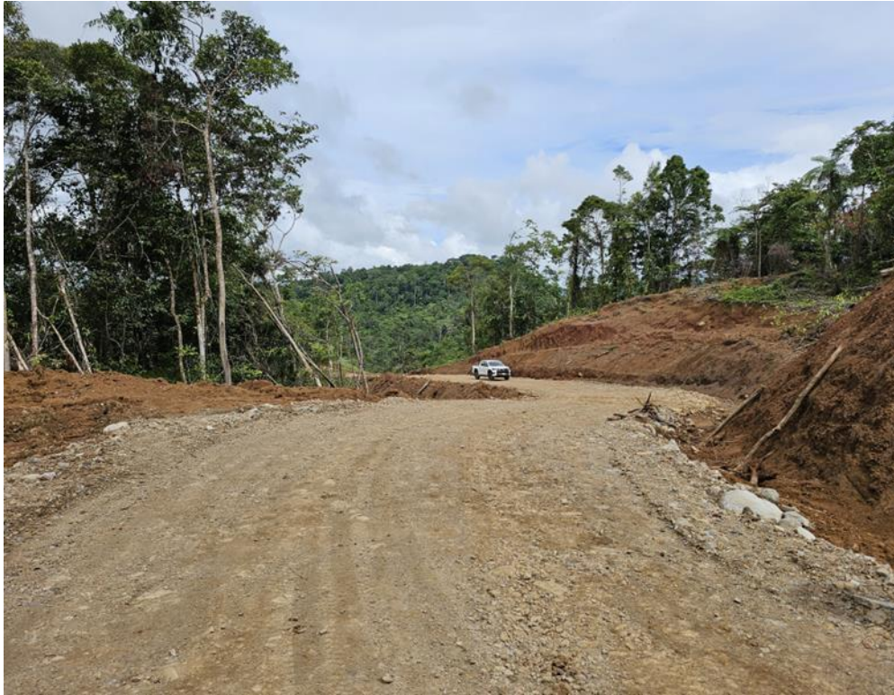
Section of the New Tolukuma Access Road
