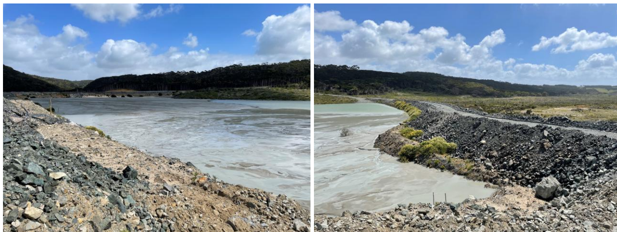
Figure 15 Tailings Storage Facility
