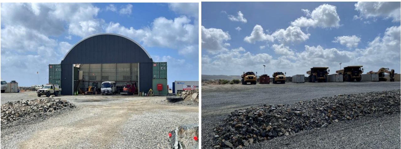
Figure 13 Workshop and Laydown area
