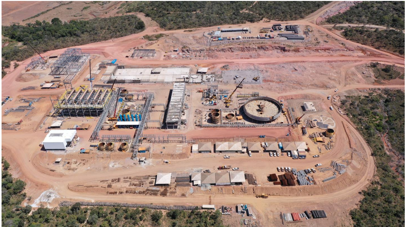
Figure 6: Serra Verde plant construction (taken in May 2022).
