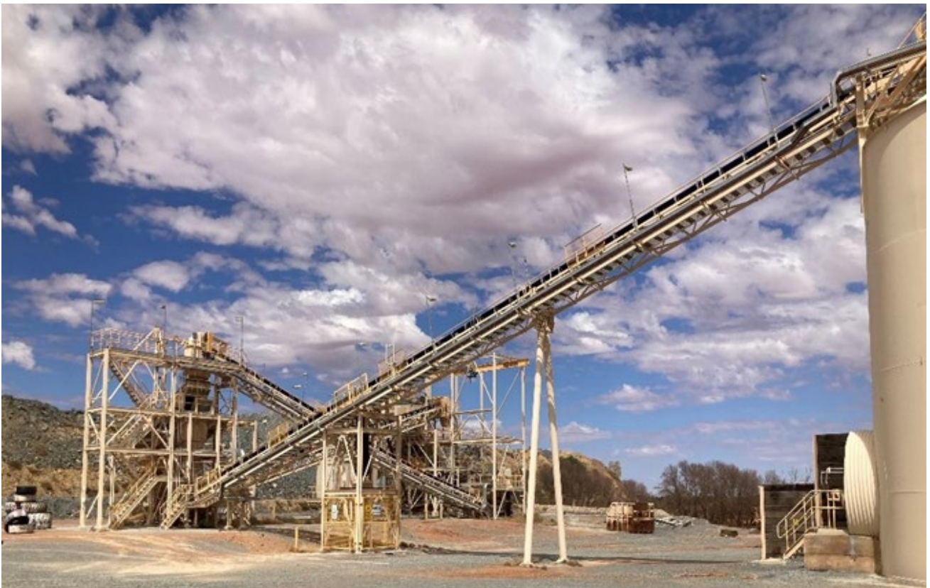
Figure 39 – View of ROM bin and crushing plant looking southwest.
