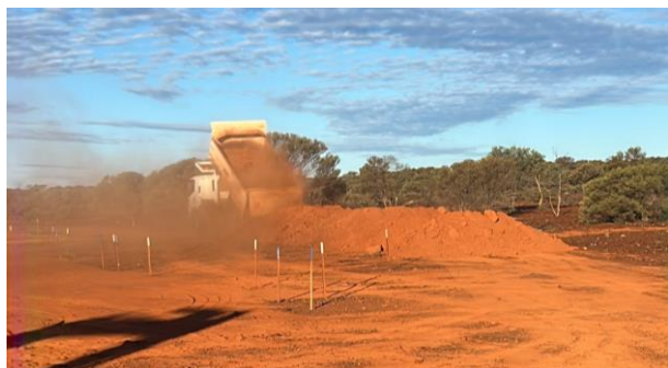
Figure 2: Preparations of foundations for administration infrastructure, July 2024.
