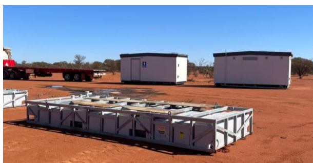
Figure 5: Buildings being delivered to site, June 2024.
