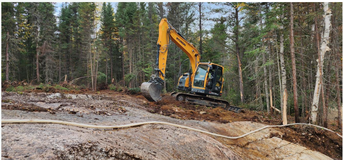
Figure 7 – Mechanical stripping of Koshman pegmatite
