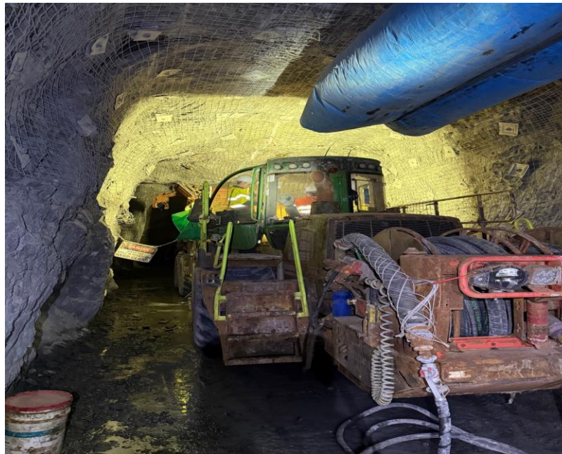
Barmingo rhino rig drilling a boxhole in the first stope to be mined at Dalgaranga
