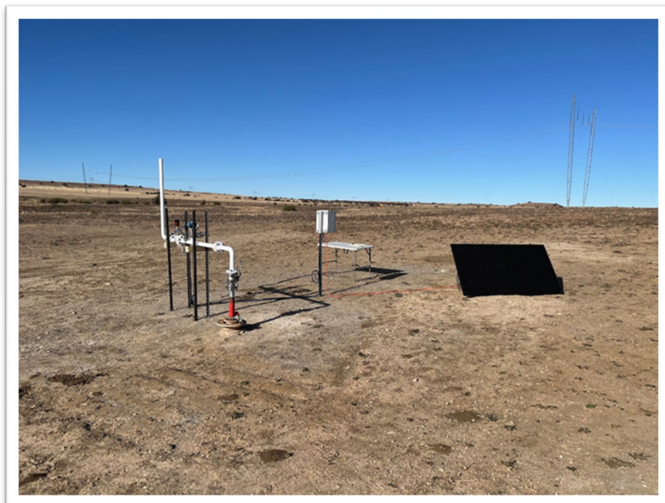
Figure 1 – new testing equipment in-situ in ER315
