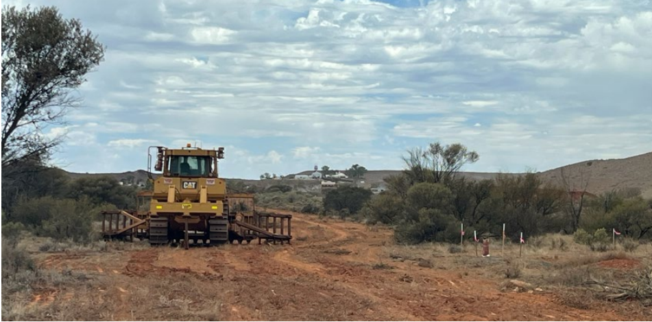
Figure 6. Tower Hill - Clearing of services corridor underway
