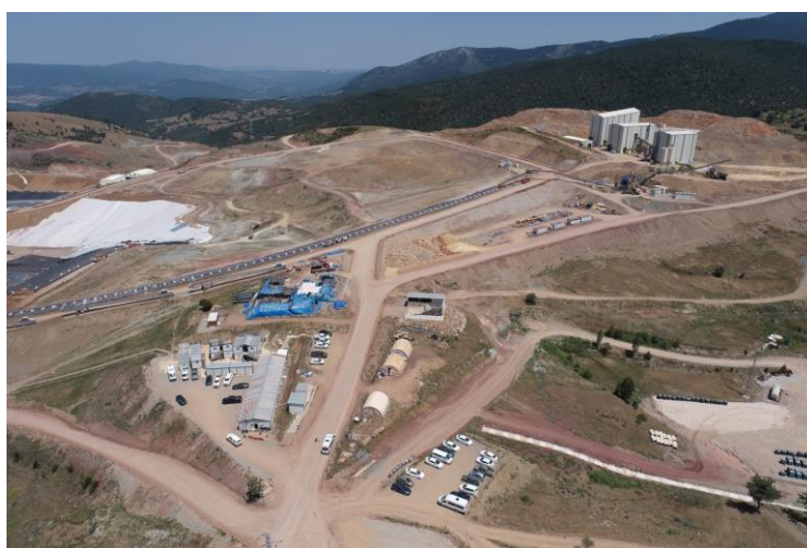
Figure 3: General site view at Tavşan showing the mine offices in the foreground with crushers, screens and agglomerator shown towards the top right. The overland conveyors to the Phase 1 heap-leach pad are installed and run diagonally across the image. Photograph taken in mid-June 2025.
