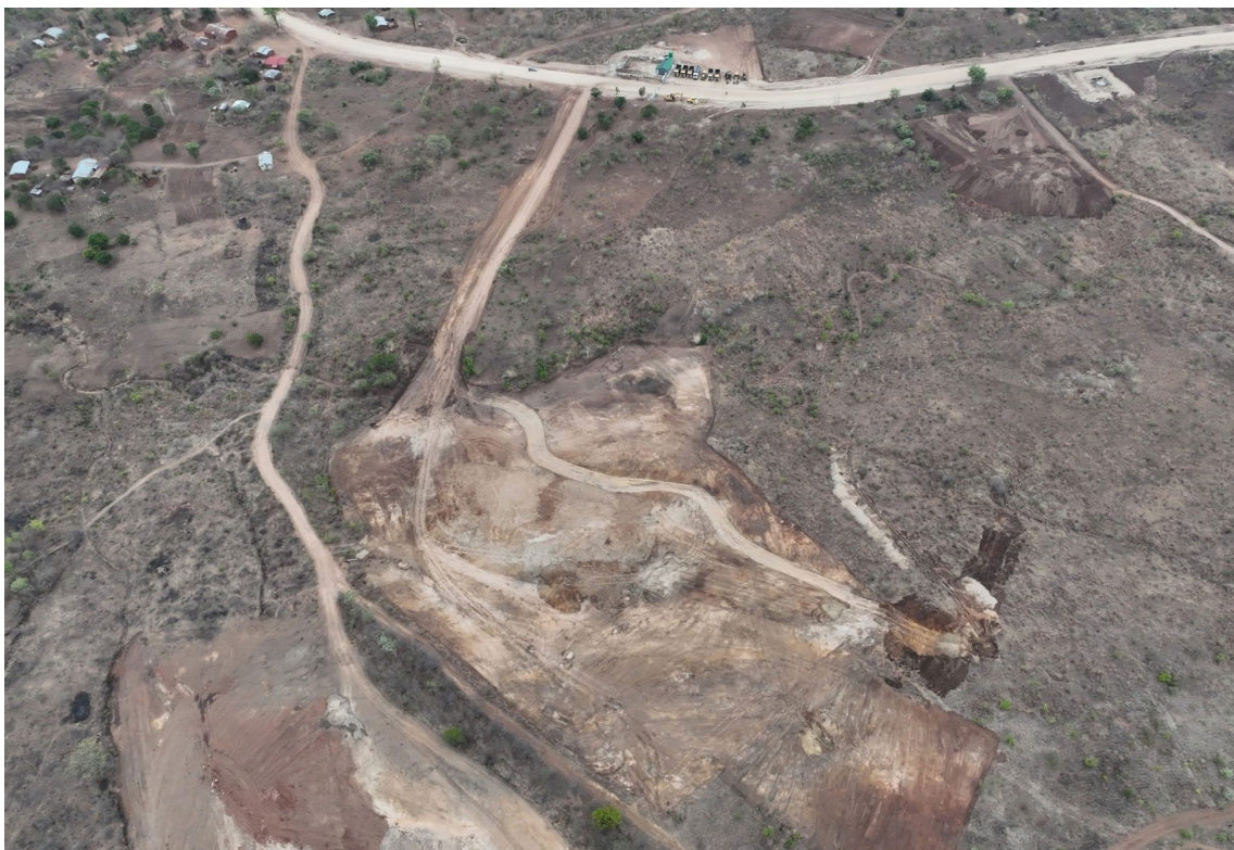
Picture 1. Clearing complete at the future Tipume Camp site at Kangankunde
