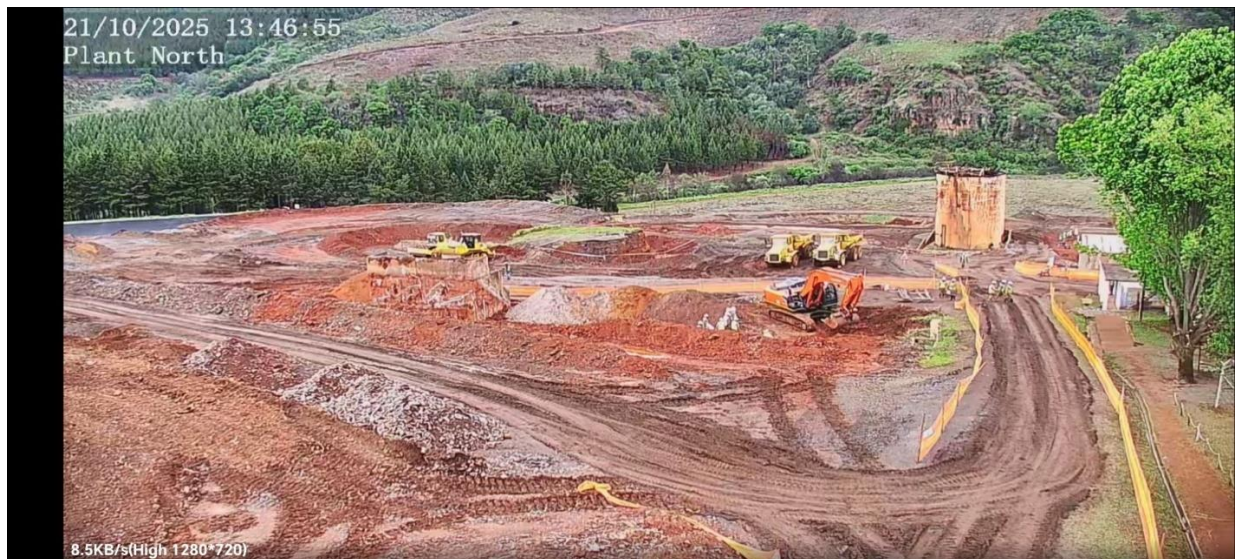
Figure 8: 21/10/2025 General Site Overview
