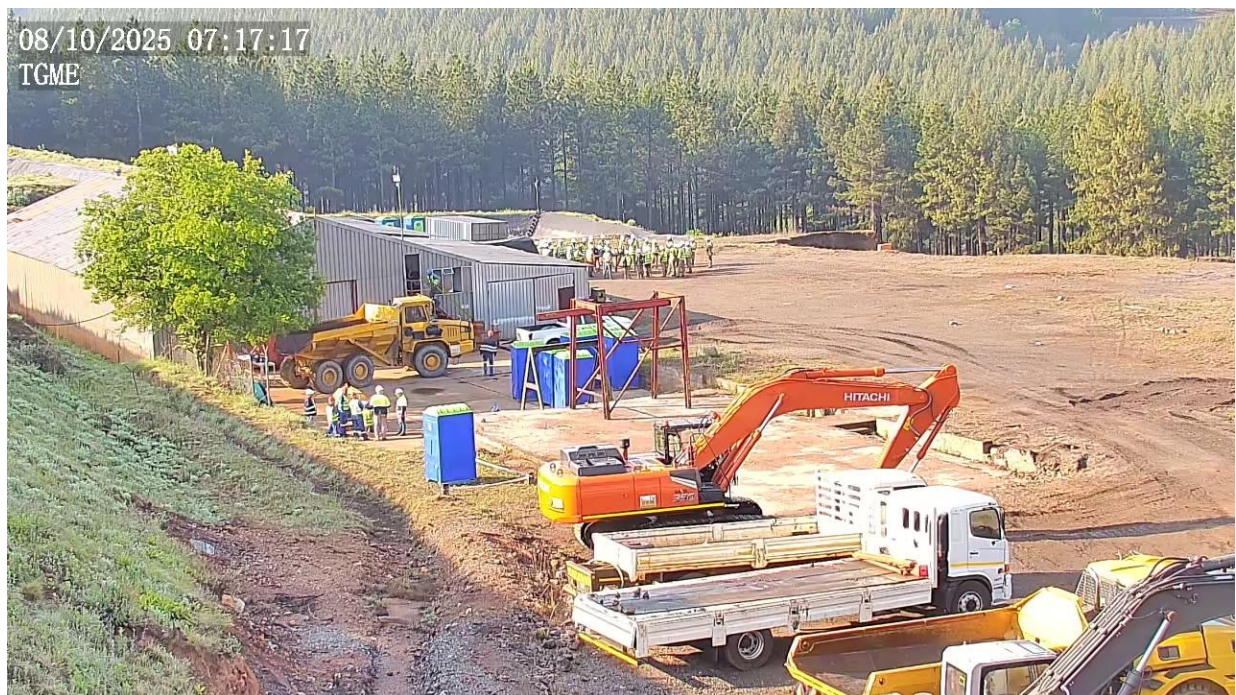
Figure 9: Safety toolbox meeting before starting work
