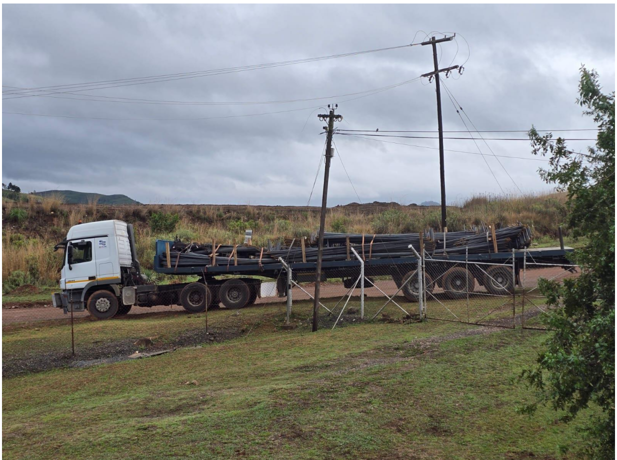
Figure 5: Steel reinforcing being delivered
