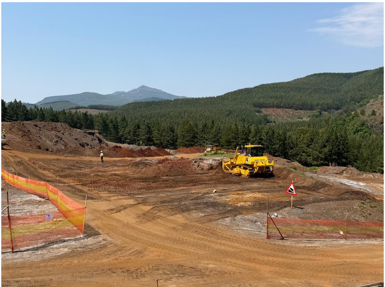
Figure 7: Earthworks on Platform 2
