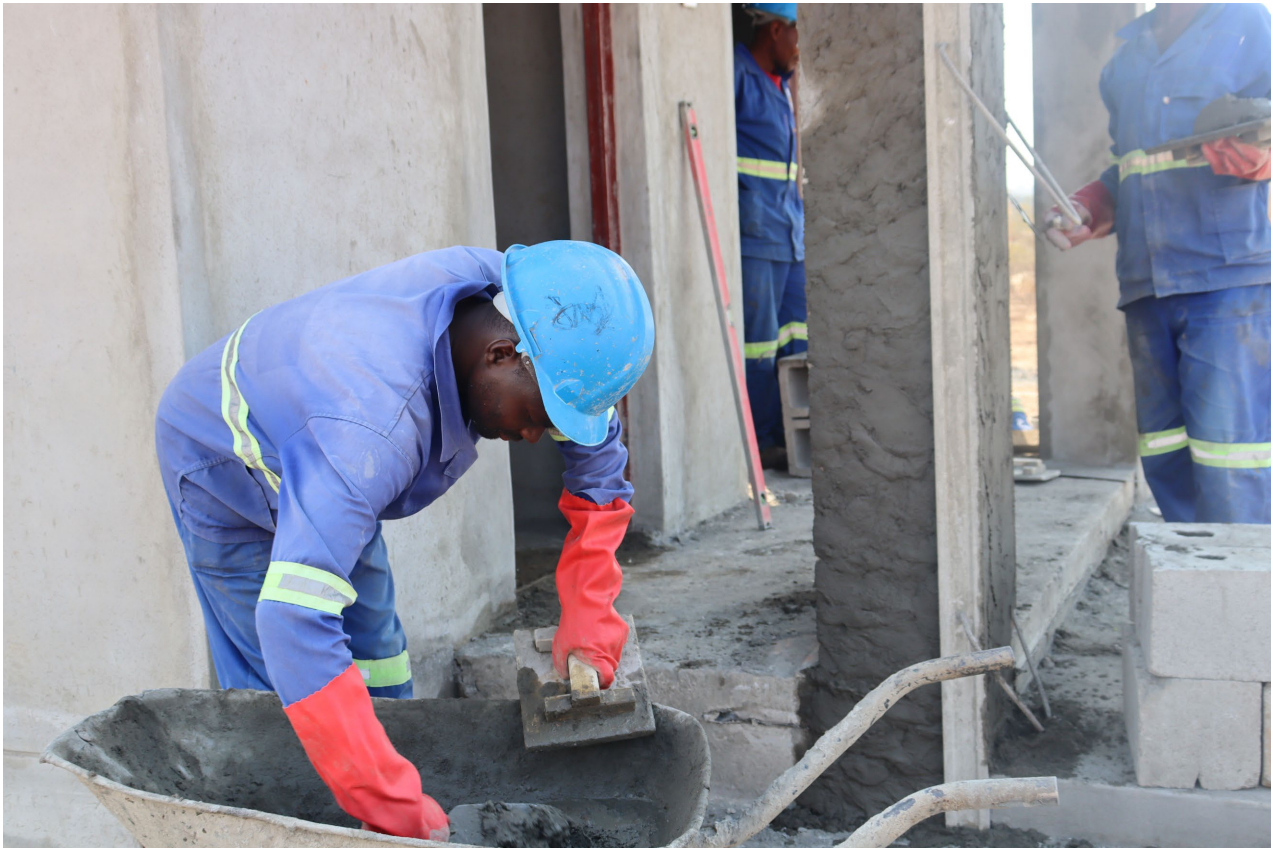
Picture 4. Employee at work on site at Kangankunde.
